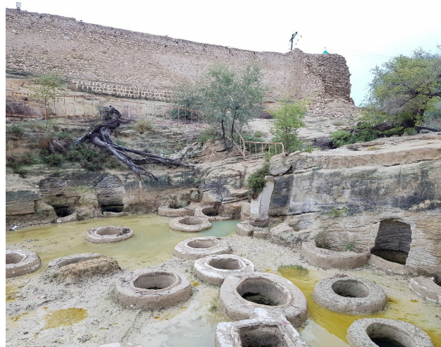
Fig. 2. "Telo"; Rainwater storage cisterns as manifestations of ecosystem service technology, Qeshm Island, Laft Port. Source: Author archive.
