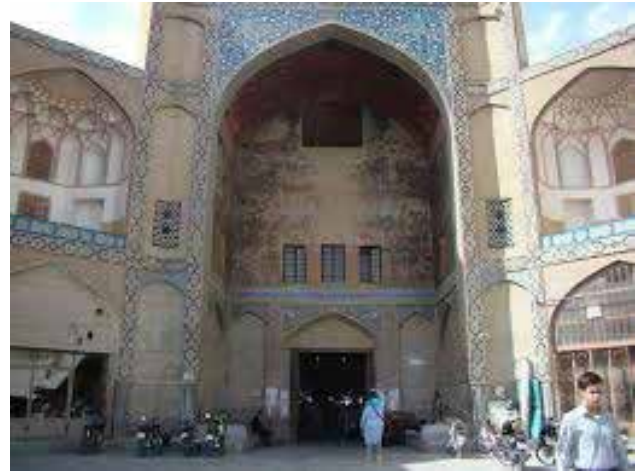
Fig. 2. The portal of Gheysariyeh Bazaar on the north side of Naghsh-e Jahan Square. Source: author's archive.
