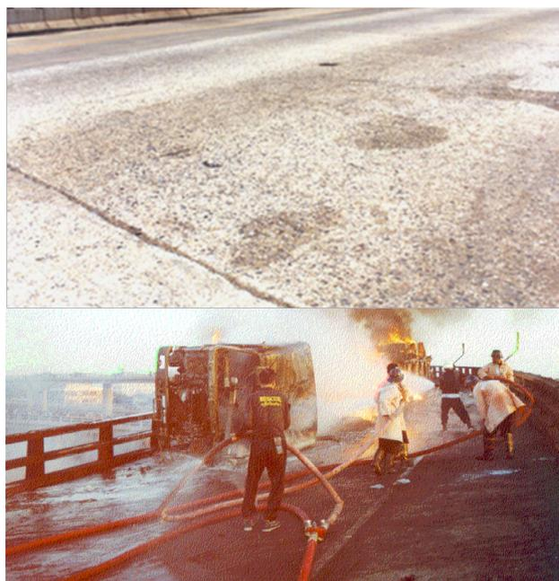
Fig. 1: Surface deterioration of concrete bridge surface due to fire and abrasion. Source: Authors.
