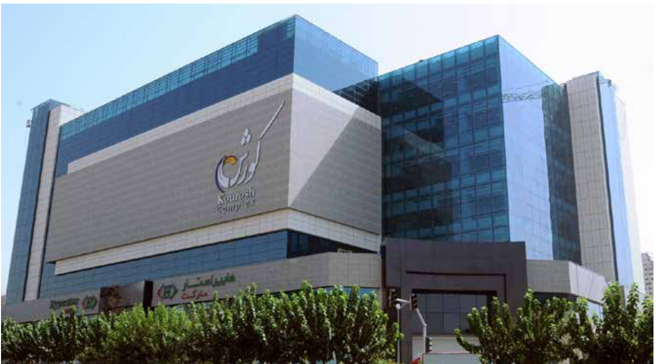
Pic3: View from outside to Kourosh Complex. Source: : http://econews.com/fa/content/1057178
