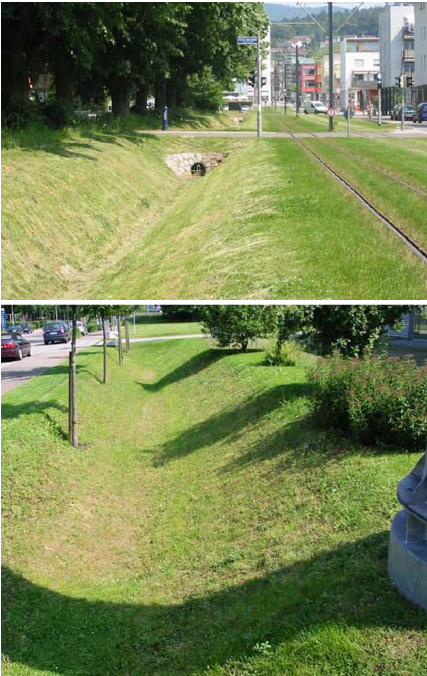
Pic 9: Stagnant pools at Vauban neighborhood; these vegetated ponds allow water to gradually seep into the soil and they supply the underground water resources. Source: http://www.hqe.guidenr.fr/images/depollution-eaux-pluviales-noue-fosse.jpg .
