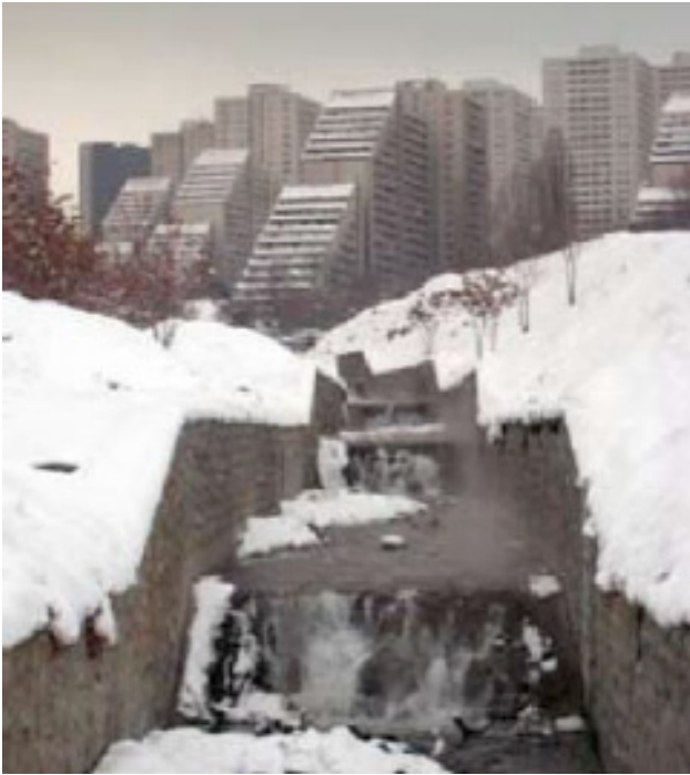
Fig. 1. Terracing and construction of channels on the river Darakeh. Source: Sabokro, 2019.
