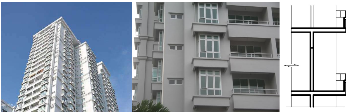
Fig. 2: Bayswater condominium of minimalist architectural style. (Left & Middle: Photos, Right: Section B B).
