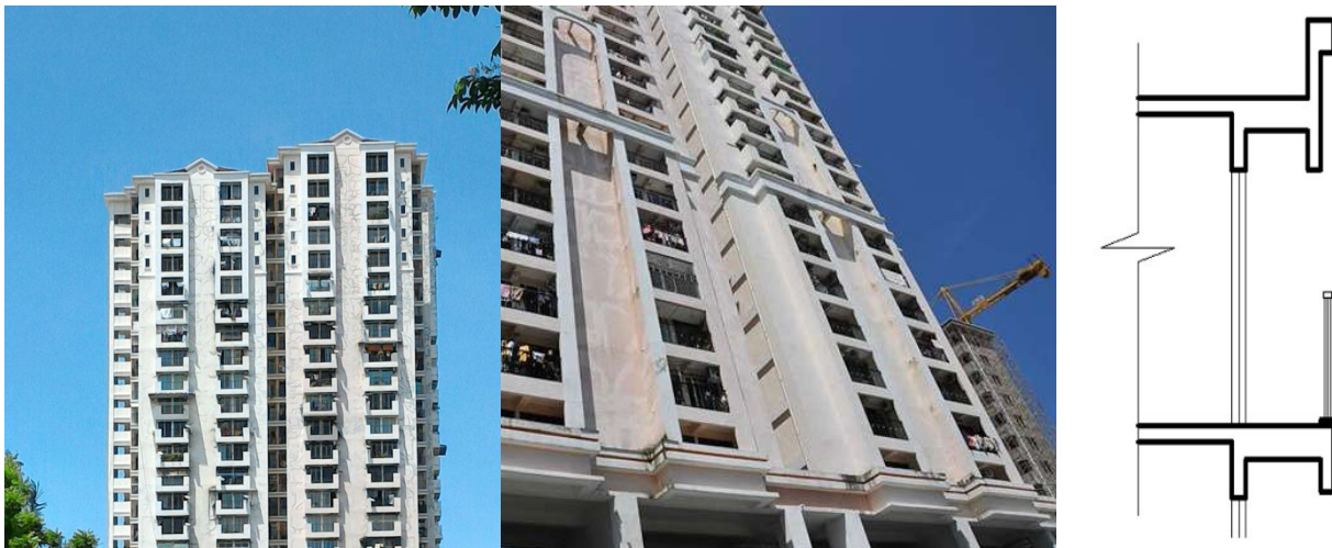
Fig. 1: Halaman Kristal apartment with colonial architectural style. (Left & Middle: Photos, Right: Section A-A).
