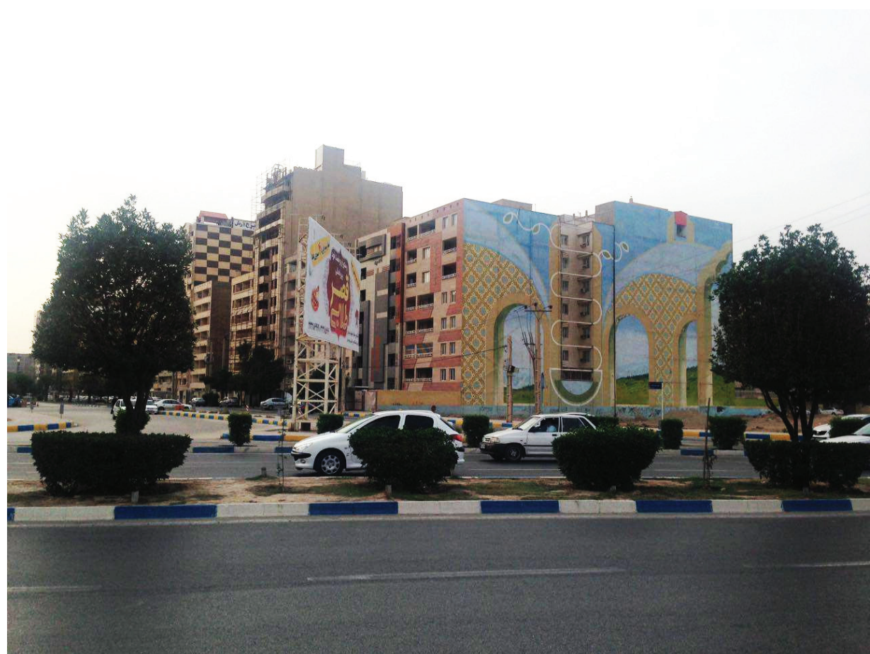
Pic 13: An example of residential buildings on the west coast (Kianpars neighborhood) that their front side has no eyelet toward the river. Photo: Morteza Hemati, 2016.
