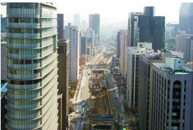
Pics 1 & 2: Cheonggyecheon River, Seoul, South Korea, during and after revitalization. Source: URL2.
