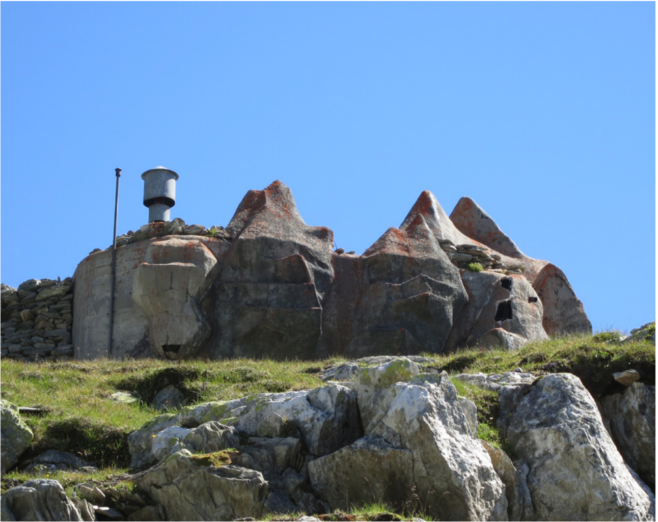
Pic 7: Switzerland is riddled with hidden and disguised military installations. What appeared to be a rock is actually a bunker made of steel and concrete painted like rock. Fortification at the Gotthard Pass. Source: https://de.wikipedia.org/wiki/Festung_Gütsch#/media/File:Gütsch_MG.JPG .
