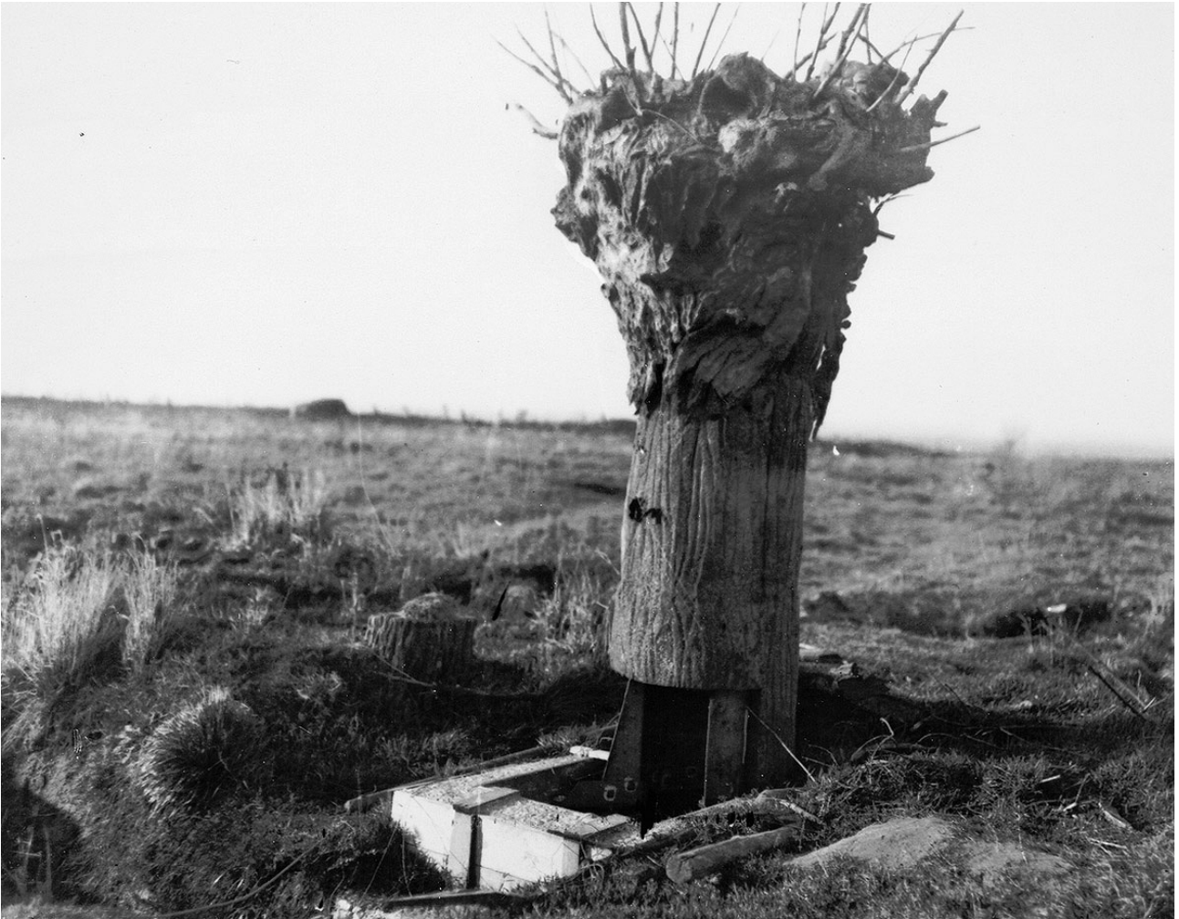
Pic 6: An artificial tree, used as a disguising observation post. Photographs and sketches of trees on the battlefield were sent to a workshop where artists constructed artificial trees using hollow steel cylinders, later installed as spy trees in the field.
