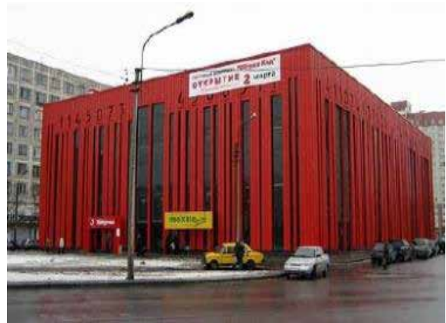
Fig. 1. Building design based on its performance (monitoring and barcode) and using warm colors in the cold and cloudy Russian climate. Source: www.apadanaart.com/fa/article , 2015
