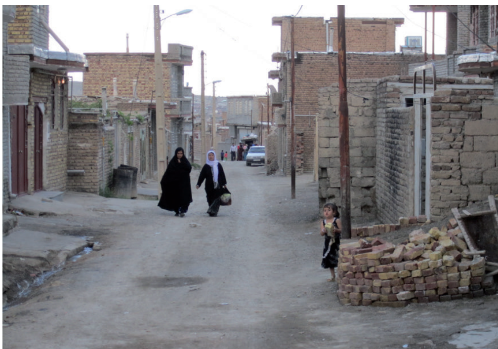
The conservation approach has forced needy habitans to migrate to other neighborhoods, Uromieh deteriorated fabric, Iran. Source: Archive of Tarh-o-amayesh consultant engineers, 2013.
